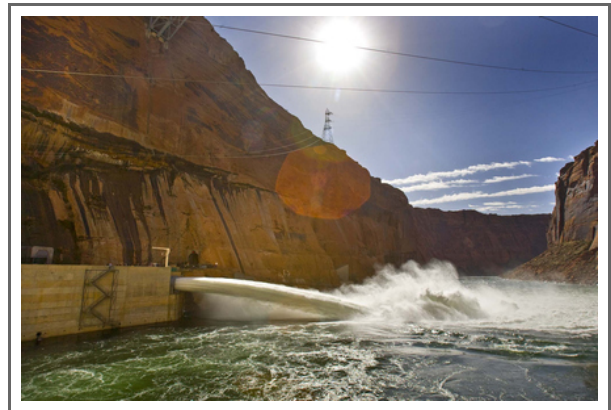
Tribune file photo Preliminary population forecasts indicate far slower population growth in Washington Canyon than previously, raising questions about the pressing need for the $1 billion Lake Powell pipeline project. In this file photo, large valves are opened at the base of the Glen Canyon Dam, sending water at a rate of 41,000 cubic feet per second into the Colorado River from Lake Powell.
